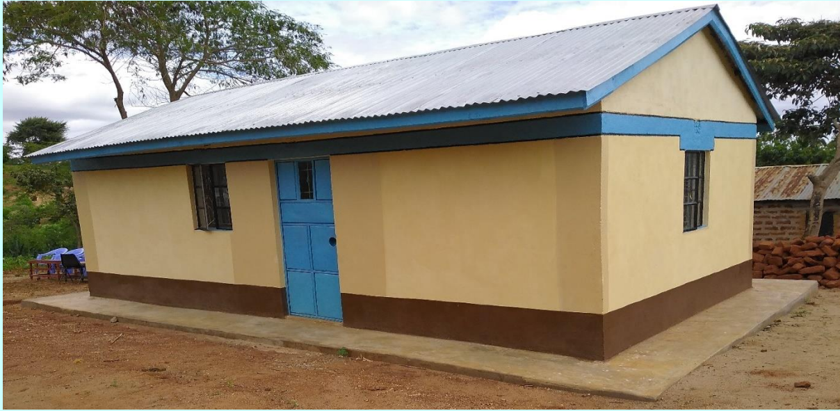
Photo 11: John Wambua's family house in Kitui constructed by KTSSC partners in 2019
