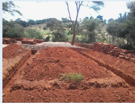
The Foundation of the Kitui House Project
