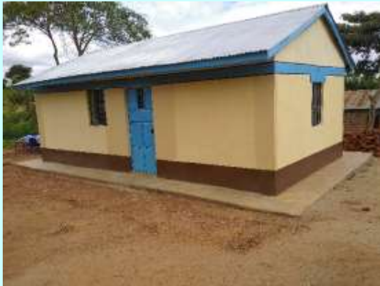
Kitui House project 2019 for Wambua's Family who is a Valter Baldaccini Foundation Beneficiary
